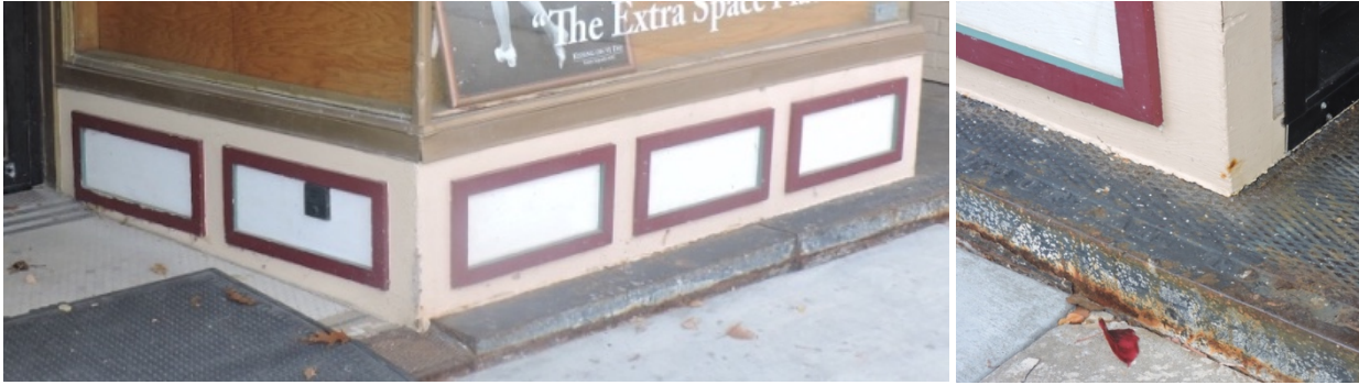
Hillmer's bulkhead is solid wood with applied panels. It is set slightly above the sidewalk on a cast iron step.
