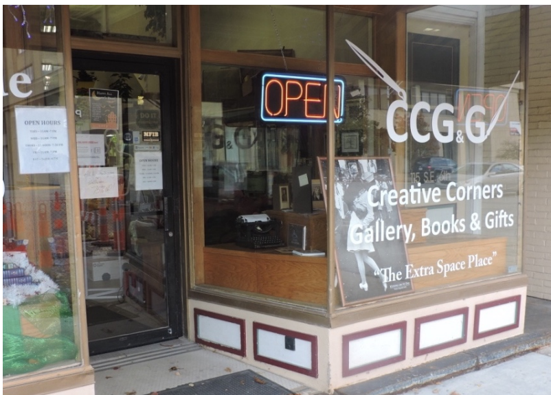
The display window at Hillmer's is comprised of large glass panels set in a thin copper frame. The painted signage on the glass enabled the current retail tenant, Creative Corners, to preserve the building's historic signage.
