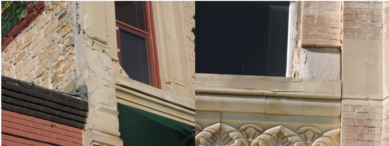
Delamination of a stone pilaster at left; spalling of a stone window detail at right.
