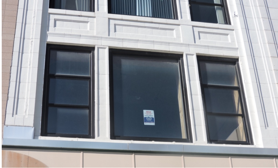
These modern replacement windows were well done, assuming that the original windows needed to be replaced due to deterioration that could not be repaired.
