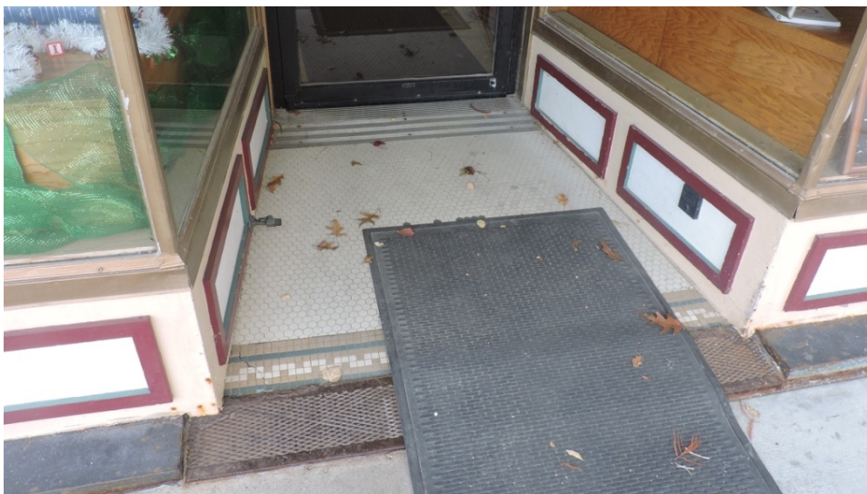
Recessed entrance vestibule of Hillmer's storefront with its decorative ceramic tile floor; the gray exterior carpet is temporary.
