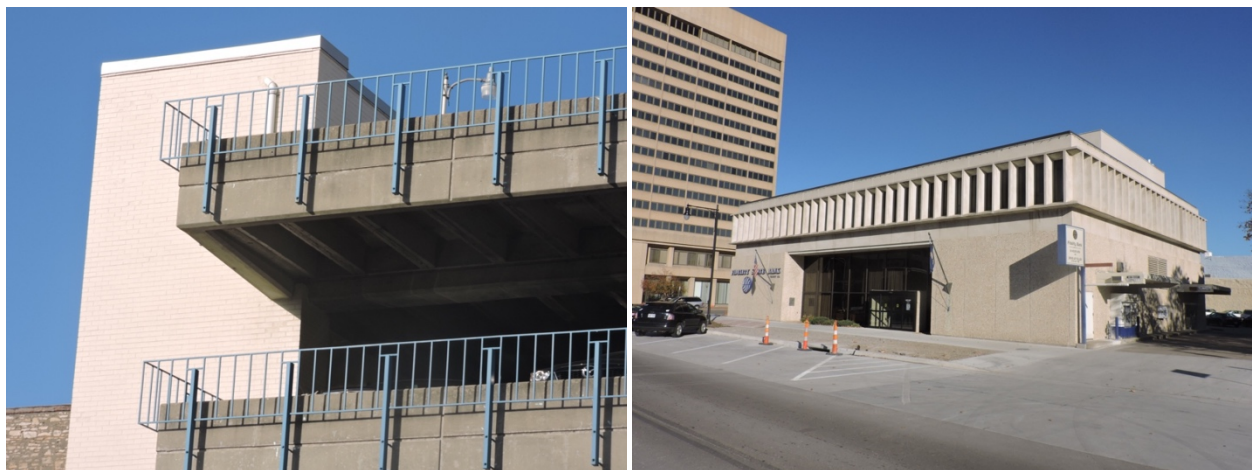
Cast-in-place concrete was used for the floor structure of the parking deck at left; precast concrete panels were used for the exterior of the bank at right.
