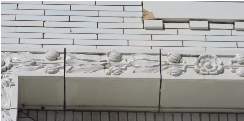
Open joints, chipping, and movement in terra cotta and glazed brick detailing.
