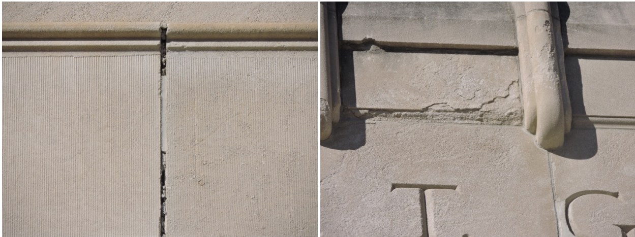
Open mortar joint and surface delamination in stone veneer walls. The open joint should be repointed. The surface delamination may not warrant repair.
