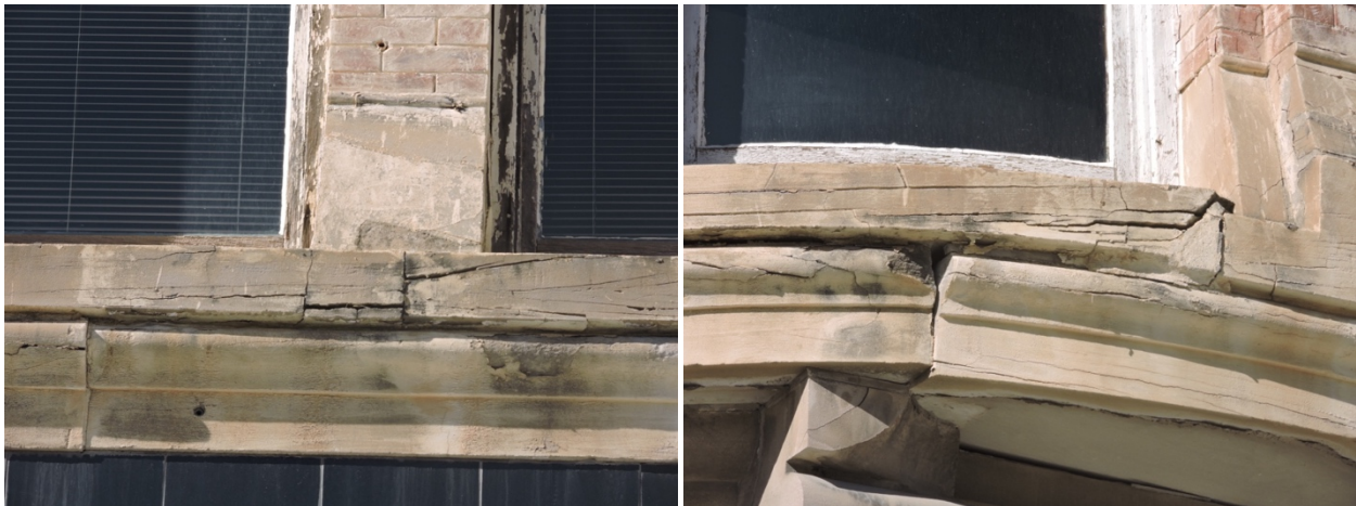
Severe horizontal cracking of stone window sills. These stones may require replacement.
