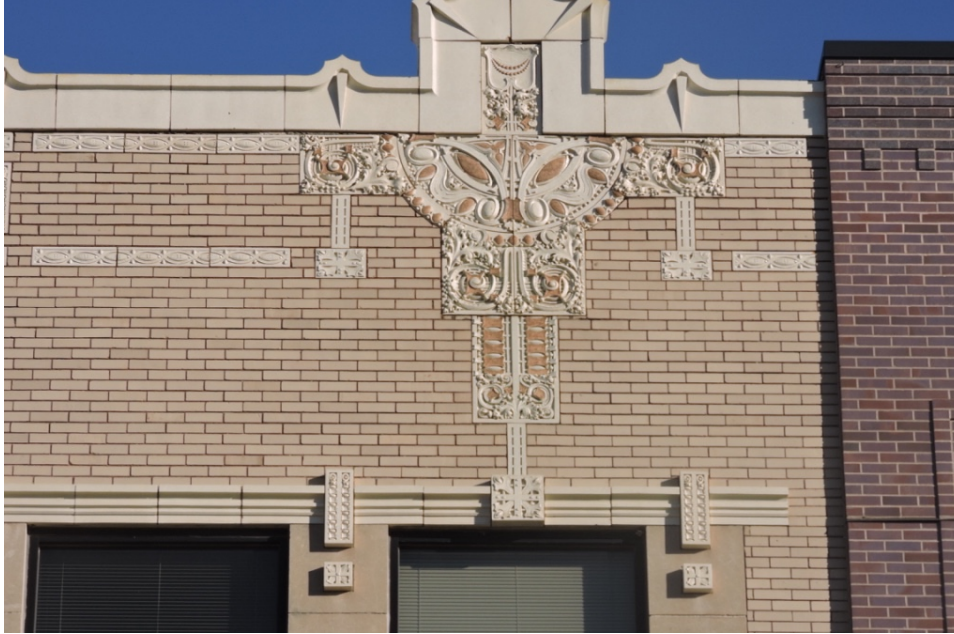
Fine terra cotta façade detailing that should be preserved and maintained.
