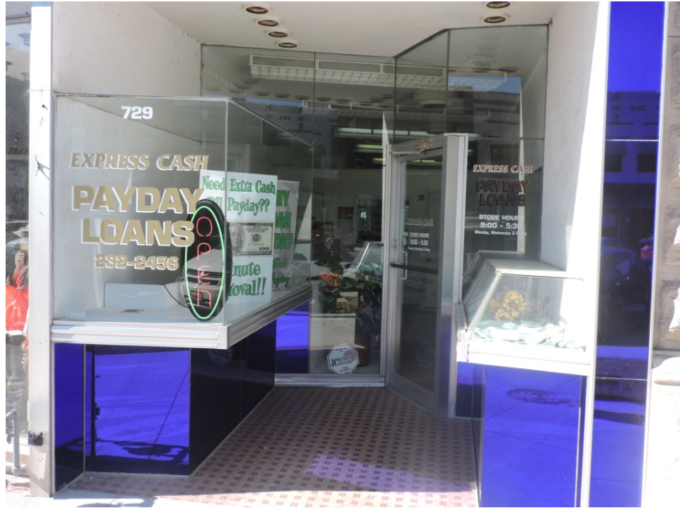
The colorful storefront of 729 South Kansas Avenue dating to the mid-1960s. The design uses reflective structural glass, aluminum, and clear display glass with sealant joints.
