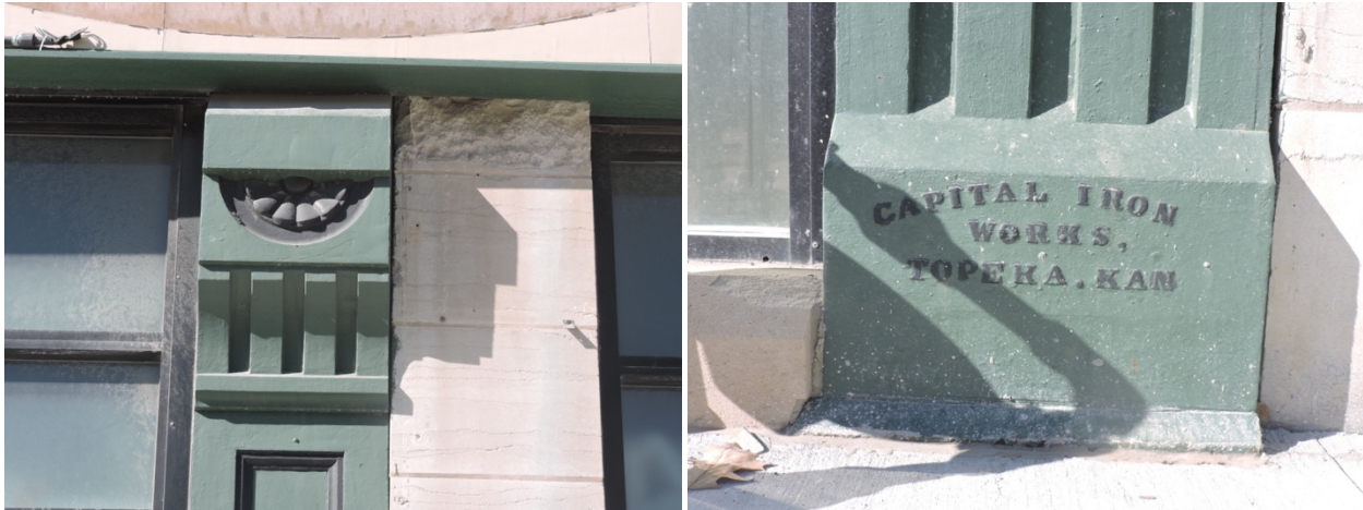
Details of cast iron column on one building; a number of cast iron columns and other elements remain.
