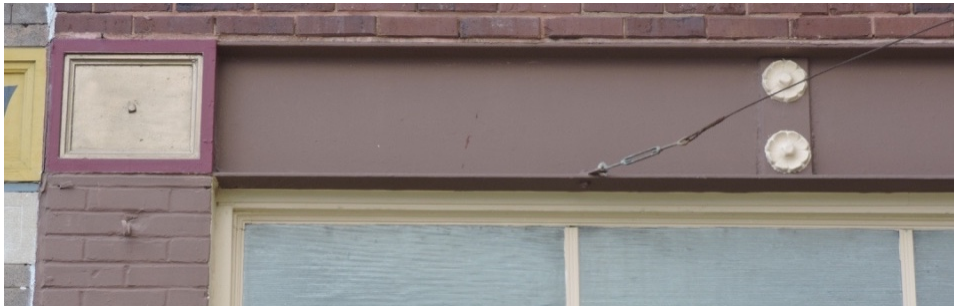
The cast iron or steel beam spanning Hillmer's storefront resting on its masonry column/end wall
