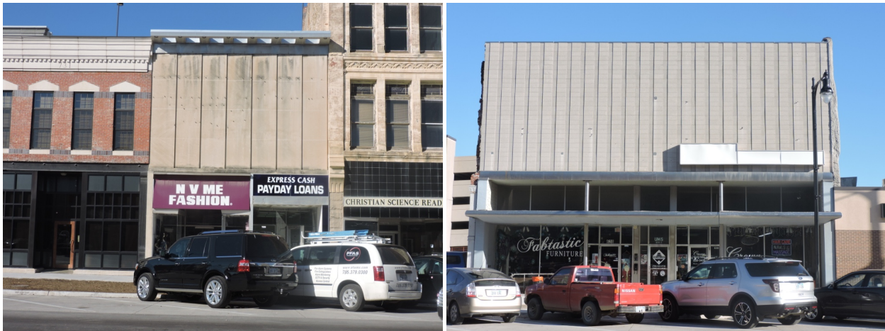
Precast concrete applied facades installed in the 1960s; each façade had large sign lettering similar to that on Briman's Leading Jewelers, pictured earlier in this chapter.
