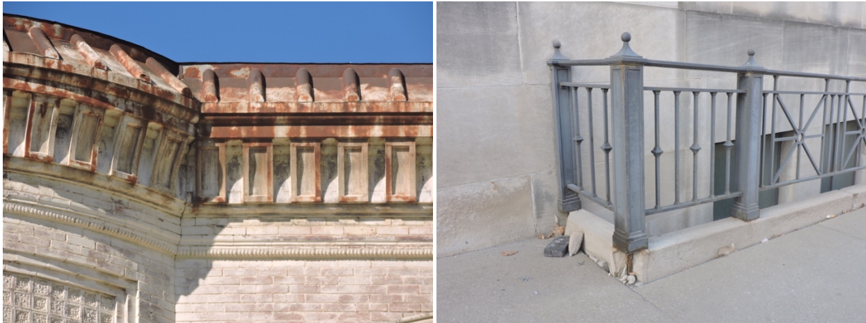
Sheet metal cornice needing maintenance at left; at right, the rusting of the base of a steel railing has expanded and fractured the concrete curb in which it is embedded.
