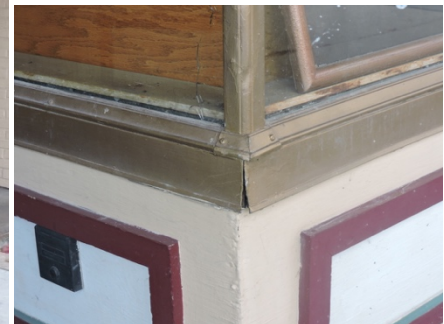
The display window at Hillmer's is comprised of large glass panels set in a thin copper frame. The painted signage on the glass enabled the current retail tenant, Creative Corners, to preserve the building's historic signage.
