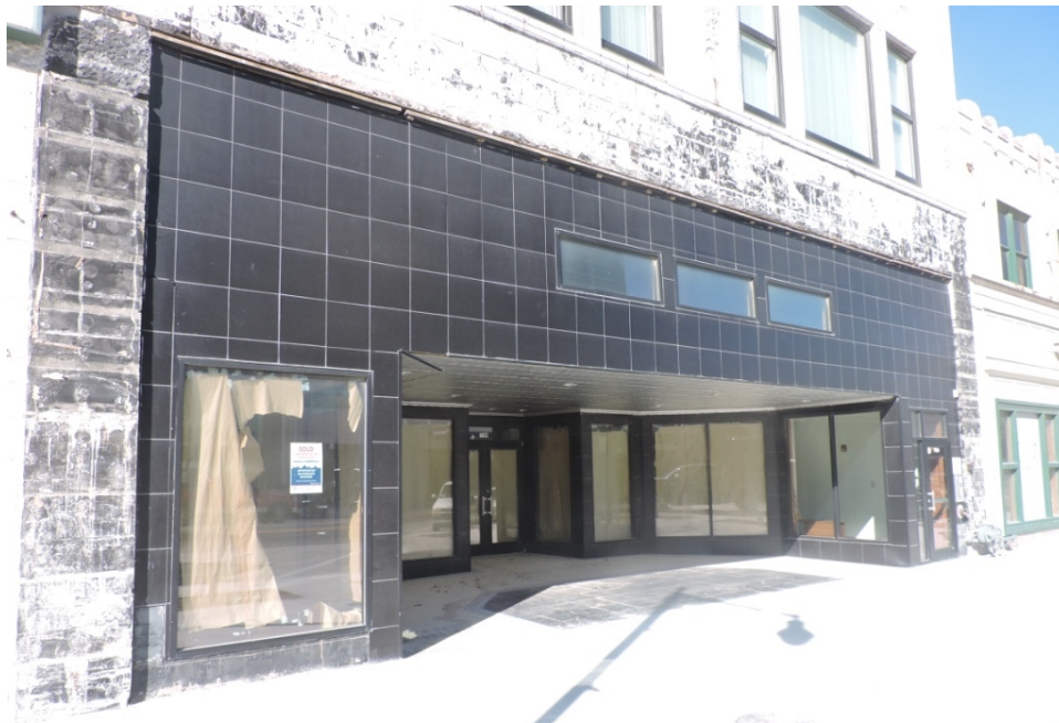
The Palace Building at 709-711 South Kansas Avenue was constructed in 1908 and altered in 1915. The black glazed tile is a still later alteration. The original building had a center display island, the footprint of which remains visible, that was removed when the tile renovations were made.
