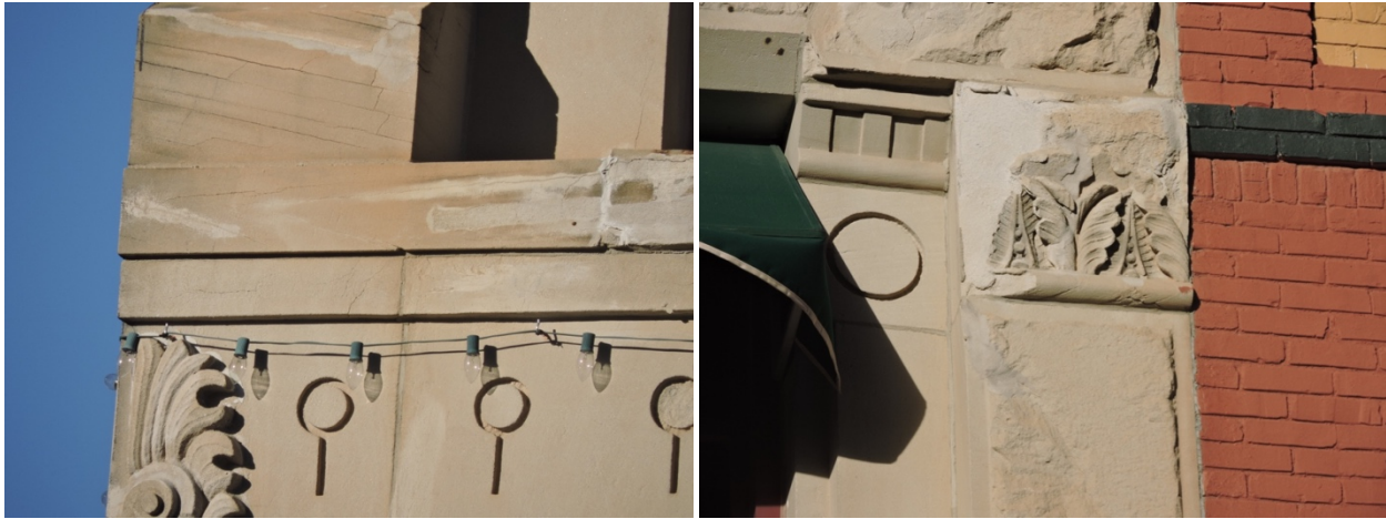
Consolidant used over horizontal cracks in stone at left and roughly over deteriorating stone detailing at right to simply prevent further disintegration.
