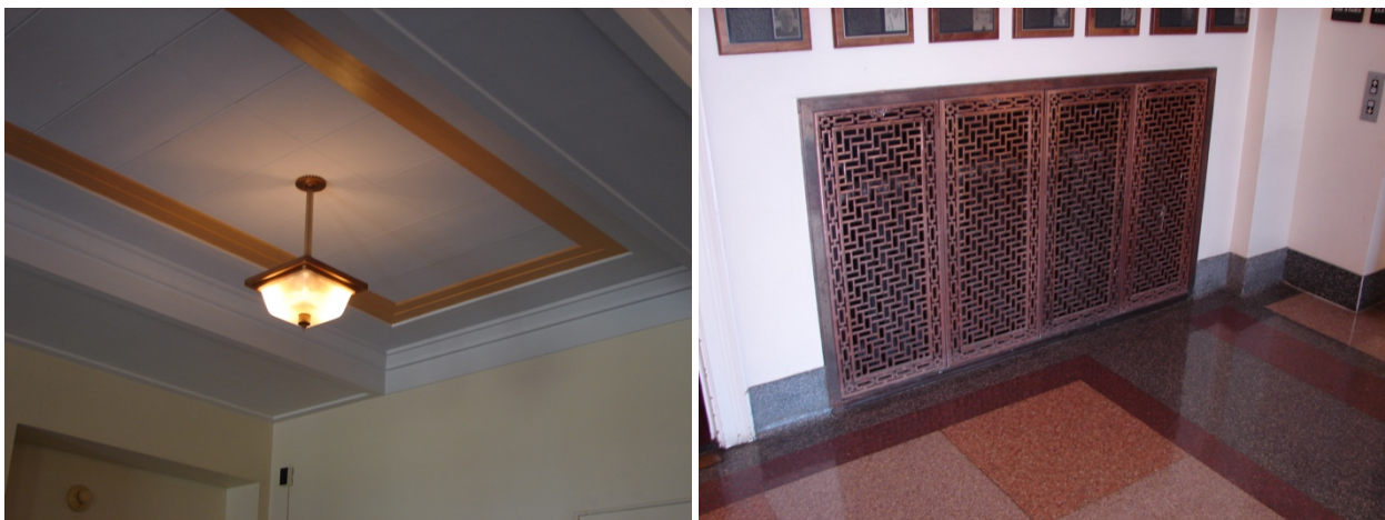
Remnant historic light fixture and heating grill that were retained in rehabilitation of public spaces.
