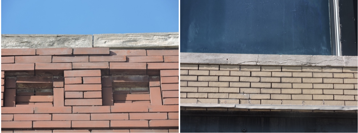
Open joints, dislocated bricks, and deteriorated stone in the walls of two Topeka buildings. The wall on the left is a building parapet; parapets are particularly vulnerable because of their exposure and difficulty to observe.
