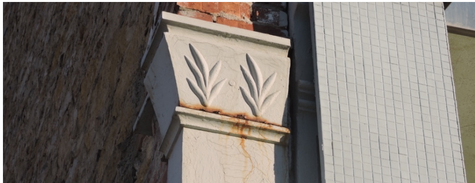
Remnant nineteenth century cast iron column encased by a later 1960s facade
