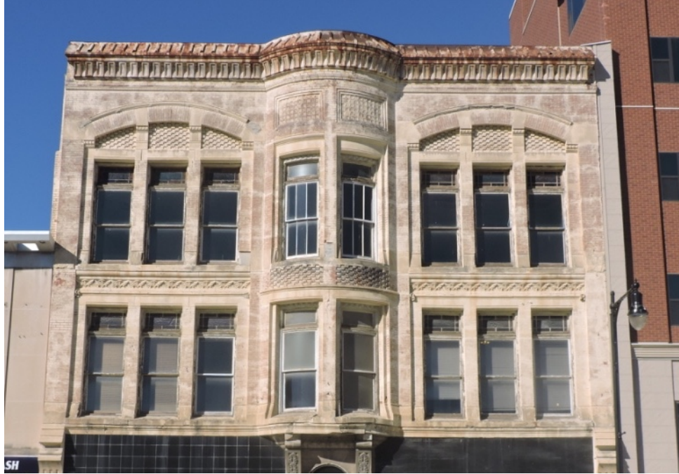
Topeka's late-nineteenth century buildings are particularly significant and vulnerable. The Davies Building, shown here, combines both brick and stone masonry with complex detailing. The bearing wall construction quality of the period was in transition.
