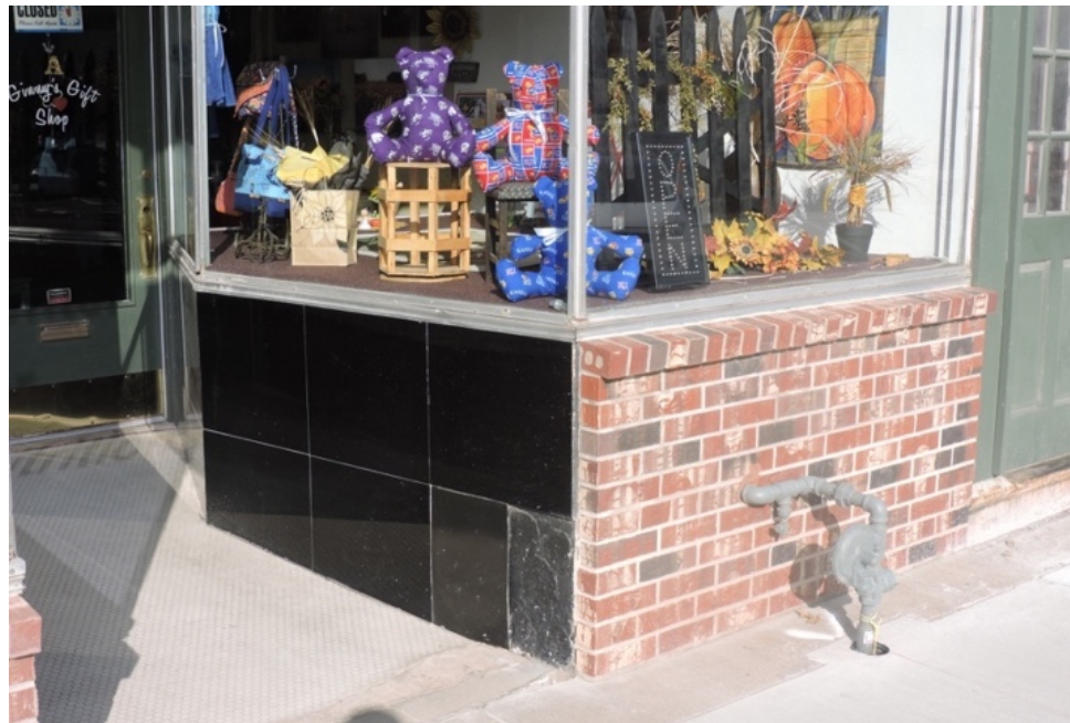
Remnant black structural glass in a storefront bulkhead that should be preserved at right.
