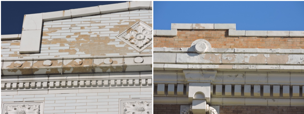
Surface delamination and spalling of terra cotta glazed surfaces probably caused by water penetration and absorption into the terra cotta behind the glaze. Parapets are particularly exposed and vulnerable.
