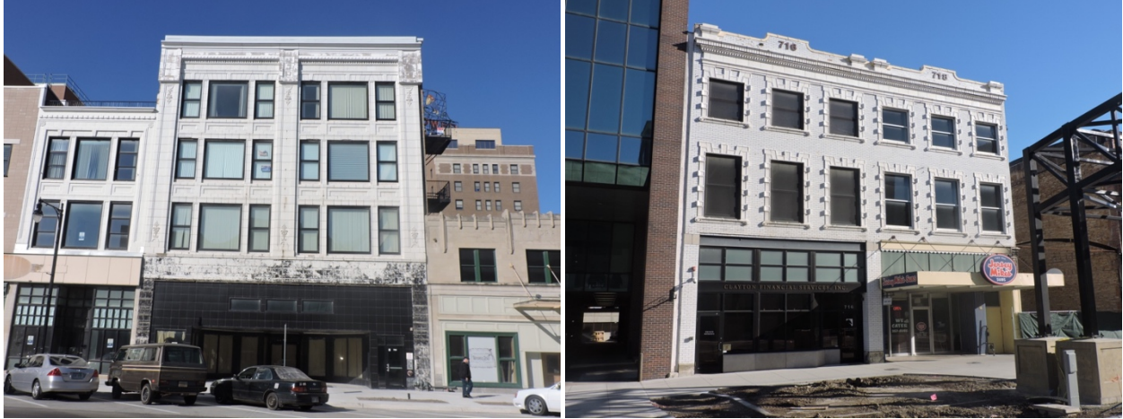
Three early twentieth century buildings with glazed brick and terra cotta facades.
