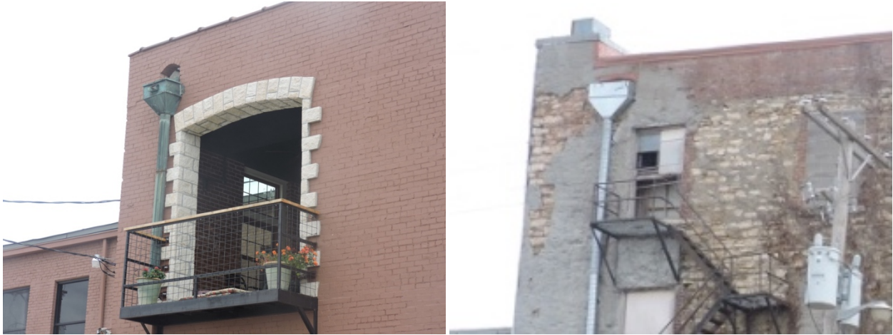
Through-wall metal scuppers and downspouts at the rear of two larger buildings. The decorative copper scupper on the left is a contributing historic feature. The rough modern metal scupper on the right is not; its downspout is probably undersized for the area of the roof it serves.
