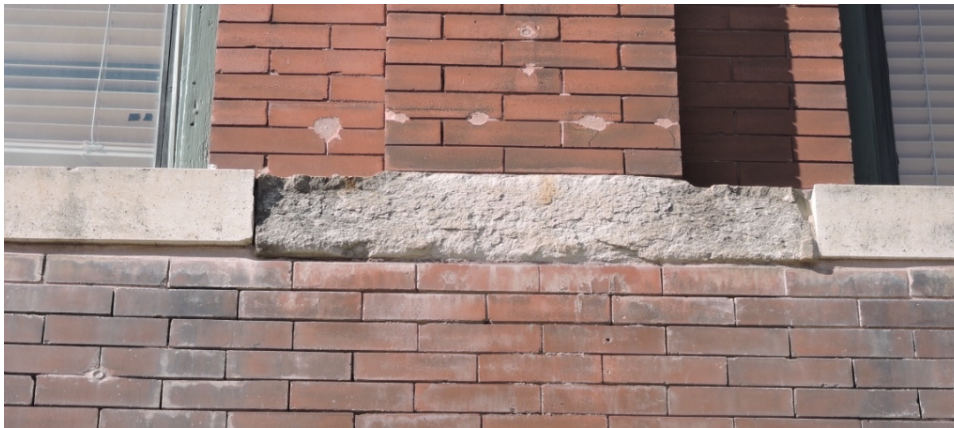
Stone sill that will require replacement.
