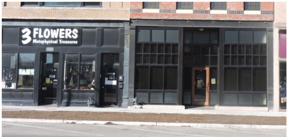
733 (left) and 731 (right) South Kansas Avenue both have cast iron beams and columns remaining. Both buildings were restored after having had their facades covered (see Chapter 2). The storefront of 733 is metal covered but recreates the spirit of its original storefront. It is possible that original wood remains beneath.
