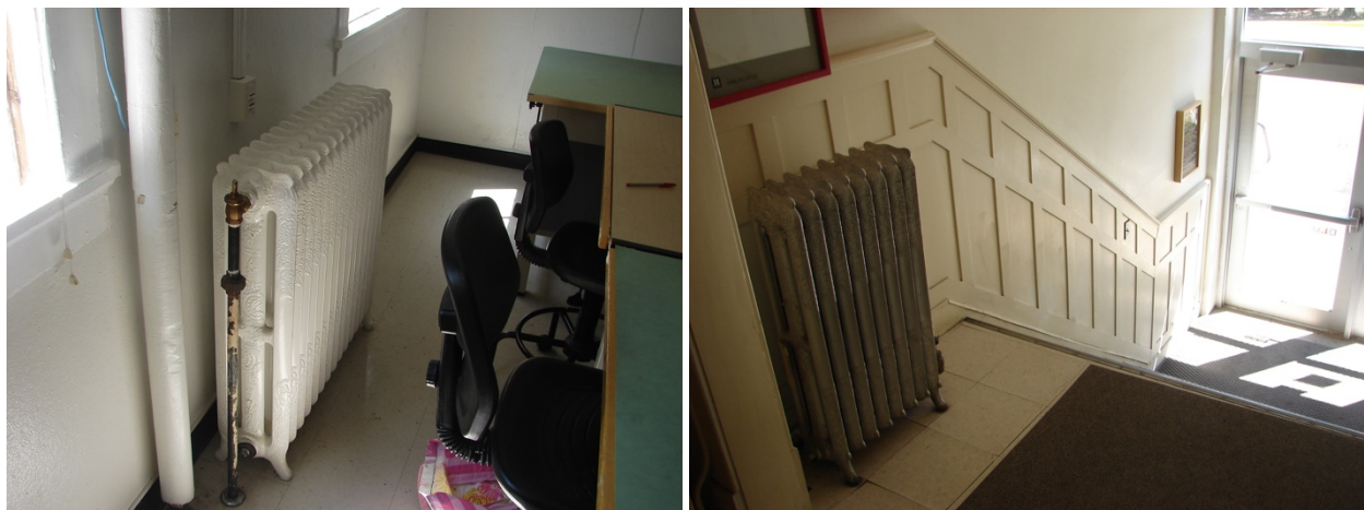
Historic radiators should be retained and can sometimes be incorporated into new heating systems.
