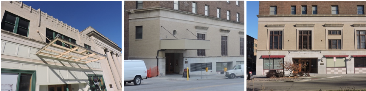
Metal frame of a canopy on Kansas Avenue; modified and missing canopies at the Jayhawk Hotel
