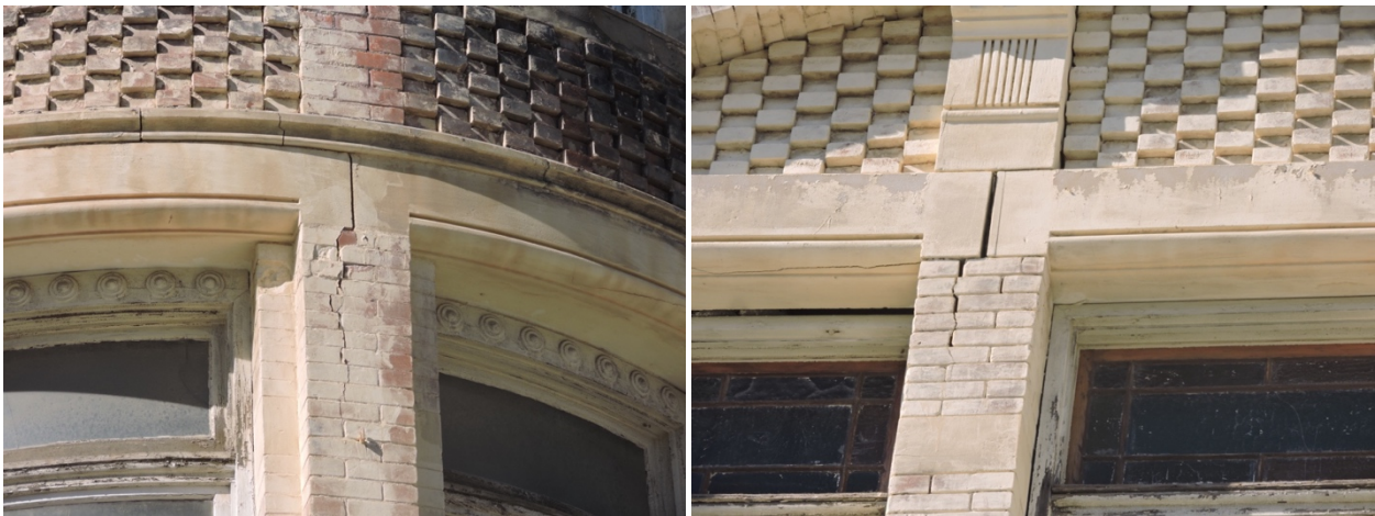
Deep masonry cracks in stone and brick piers at the Davies Building.
