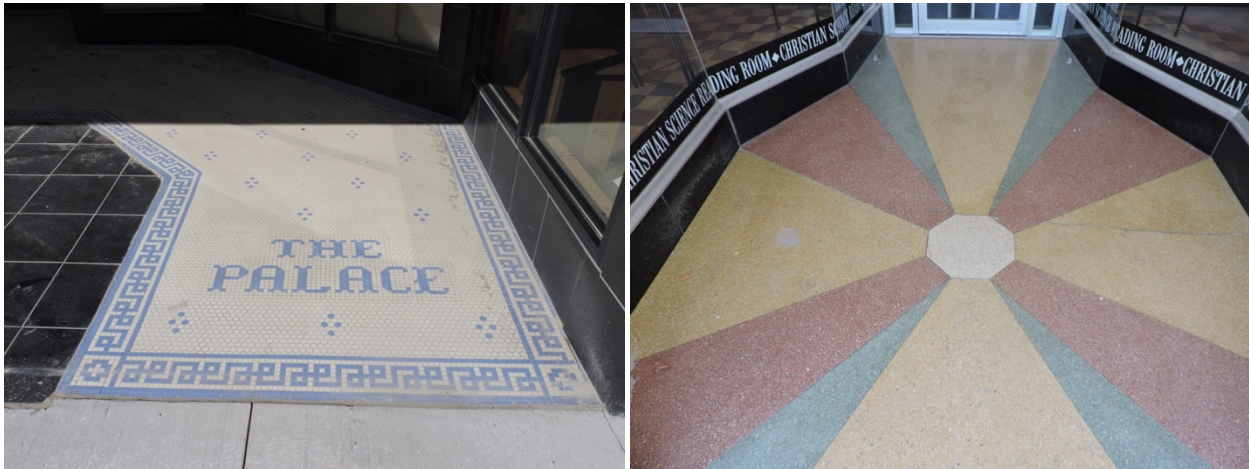
Tile storefront entrance vestibule from about 1908 on the left; terrazzo flooring in a storefront vestibule possibly from the 1950s on the right.
